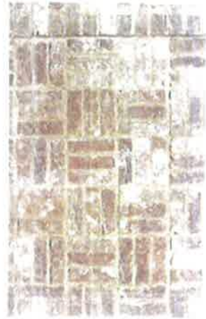
BASKETWEAVE BRICK DETAIL NO SCALE
